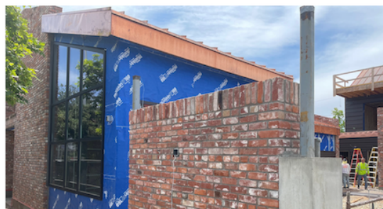
Final construction underway.
