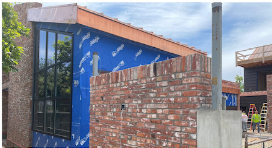
Final construction underway.
