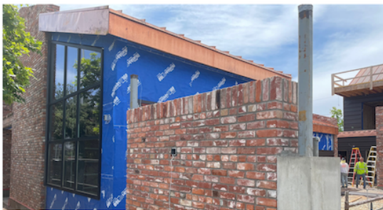
Final construction underway.
