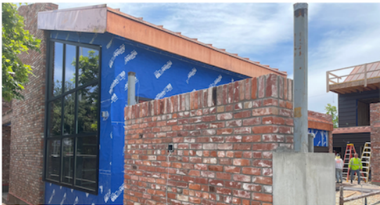
Final construction underway.
